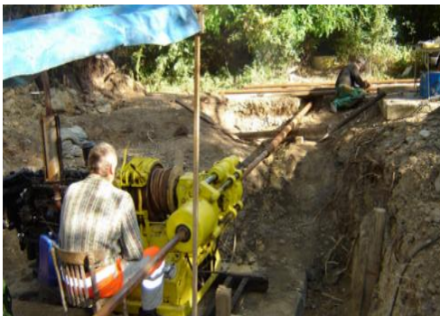
Horizontal drilling through which water will flow from the slope
