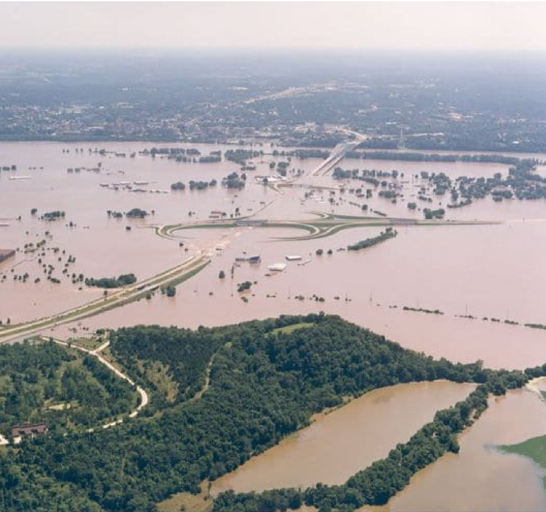
the Missouri River flooding on July 30, 1993, in the vicinity of Cedar City and Jefferson City Memorial Airport north of Jefferson City, Missouri, looking south (photograph from the Missouri Highway and Transportation
